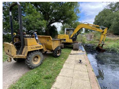
silt removal at The Wharf
