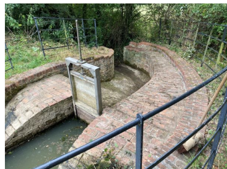
the Horseshoe Spillweir after clearing vegetation
