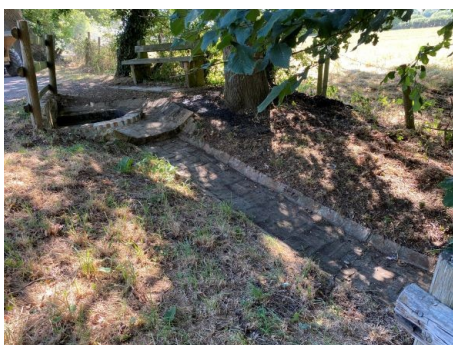
the Small Circular Spillweir after replacing brickwork
